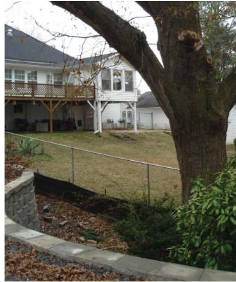
Figure 7. Undersized Tree Well
