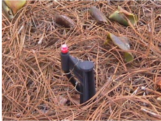
Figure 4-8. This is a micro-spray applicator positioned above a mulch layer by a plastic stake driven into the soil. Micro-sprays and micro-sprinklers must be above the mulch layer so that the mulch will not inhibit their water spray or sprinkling pattern.
