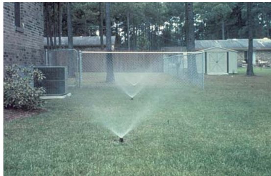
Figure 4-4. Spray applicators are pop-up style heads that will let the applicators recede below the turfgrass when irrigation stops.
